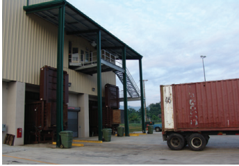
This transfer station, located in Salem, VA, features two BlokPak 3000 compactors for non-stop processing as well as added redundancy. They are fed from a tipping-floor.
